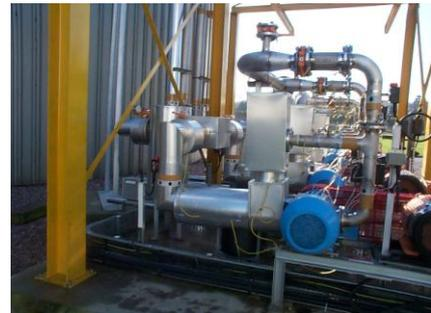
Hartshill STW operating 2No. Duty standby air-cooled oil lubricated Utile Model L240HP Gas compressors that replaced "hook and claw" type.
