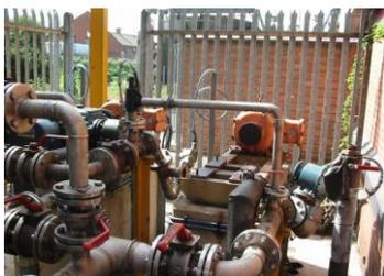
Redundant oil free compressor – replaced with oil lubricated at Loughborough STW
