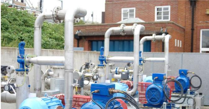
16 Utile Gas Compressors installed at Minworth STW, replacing oil free machines.
