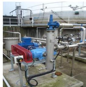
Utile oil lubricated compressors replacing oil free at Barston STW
